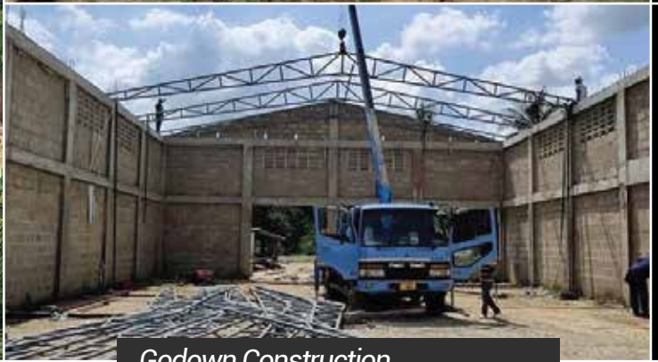
Godown Construction Dakawa - Morogoro
